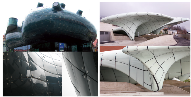
Figure 2: Projects involving double-curved panels where a separate mold has been built for each panel. These examples illustrate the importance of the curve network and the challenges in producing architectural freeform structures. (Left: Peter Cook and Colin Fournier, Kunsthau, Graz. Right: Zaha Hadid Architects, Hungerburgbahn, Innsbruck.)
